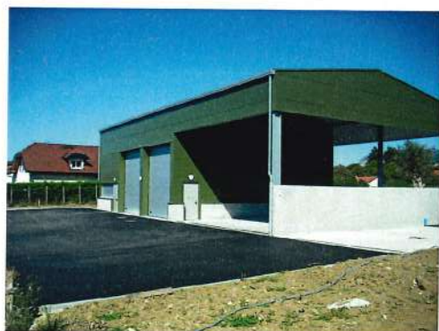
Le hangar technique communal
